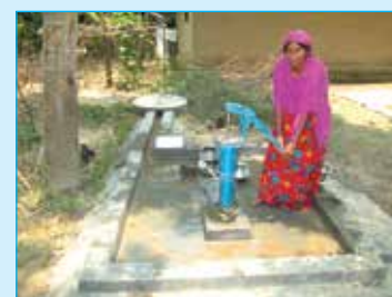
Photograph 6: Tube well installation
