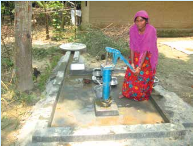
Photograph 14 : Installation of deep-set tube wells
