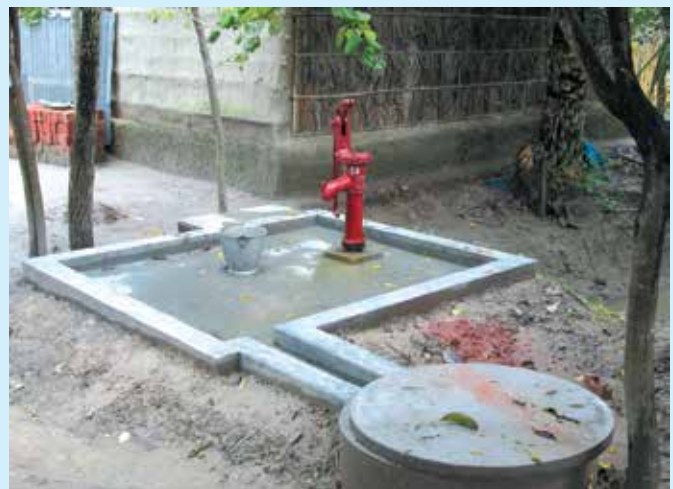
Photograph 13 : Construction of tube well platforms
