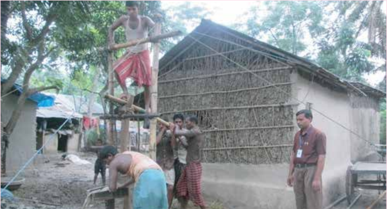
Photograph 18 : Tube-well installation in Kasharigacha Village
