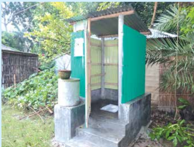
Photograph 12: Installation of Sanitary latrine
