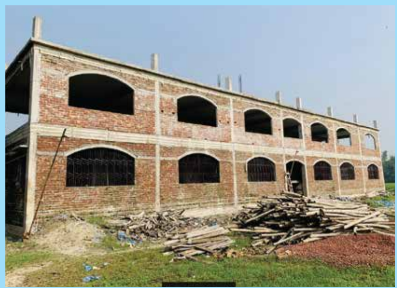
Front view of NDP Loom Training Centre (under Construction)
