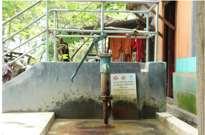
Double platform tubewell installed in Alo Khatun's house
