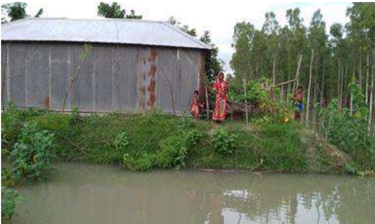
Flood recovery response program through HH plinth rising and present Flood situation at Shilpi Bagum, WBA-0073, Village-
