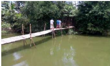
Role of VDC Bamboo bridge construction ChouhaliUpazila. Date: 11/08/20
