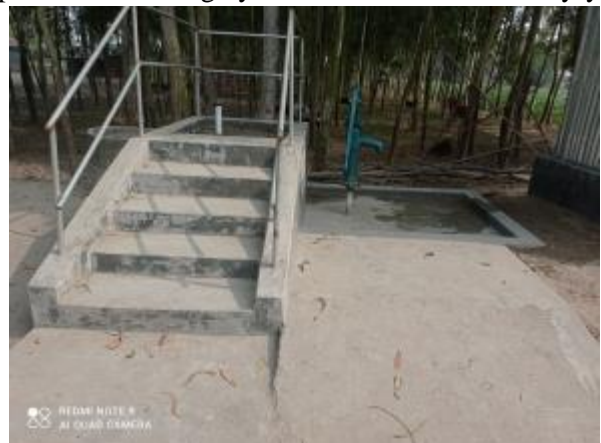
Double Platform Tube-well in UttarBurungi
