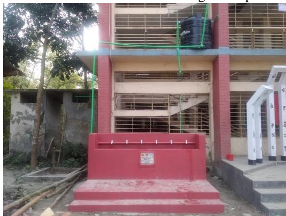
School Block Hygienic Station in Takani Union, Kazipur
