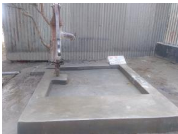
Rehabilitation Dysfunctional Water Points in Rehaishoriber
