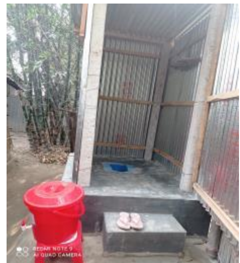
Emergency Latrine in Perkhukshia Village
