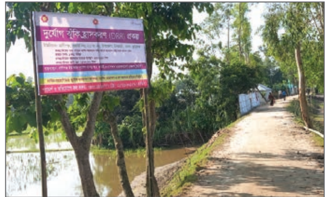
Road construction under WFP-DRR Project
