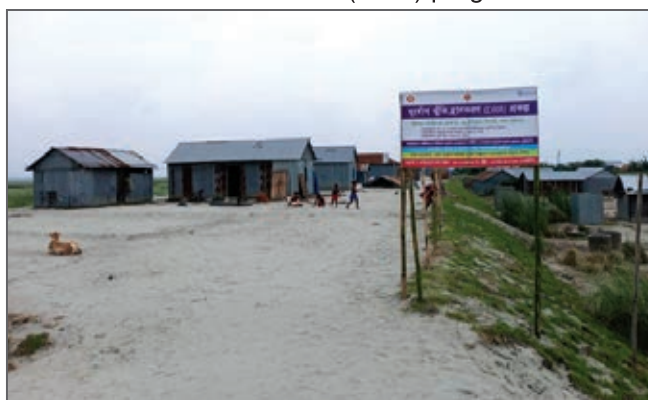
Homestead land raised under the DRR project to combat flooding
