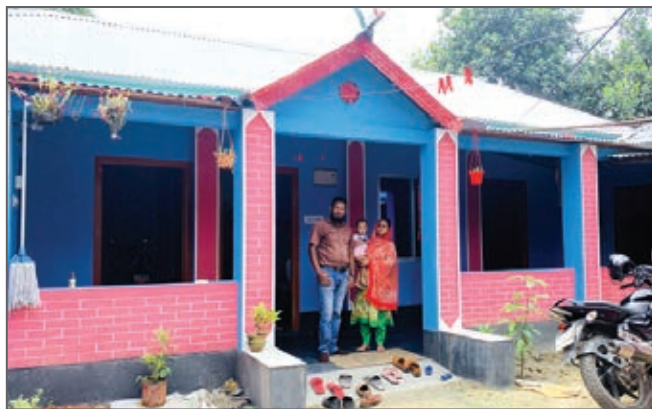
A new dream home handed over to a programme participant under the LICSHSP initiative
